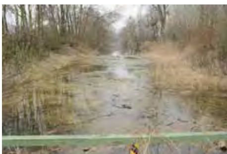
Picture 6.3: e - channel paralalel to Danube, bridge
