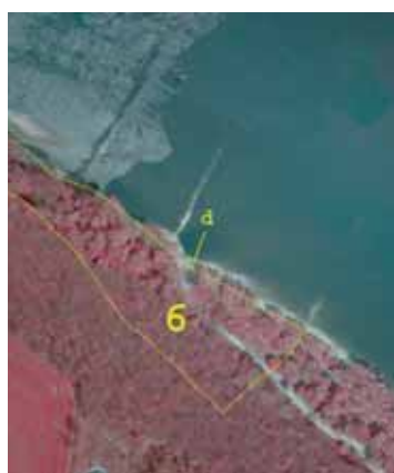
Picture H3: missing dam, water flows into the armlet
