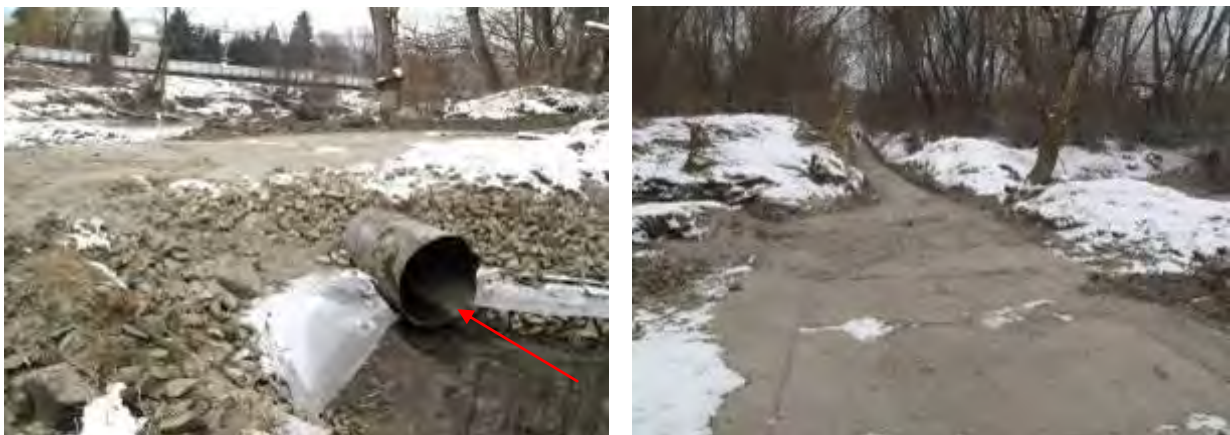
a) b) Fig.14 Interconnection of the distributary through a pipe culvert – upper part (a) roadway (b)
