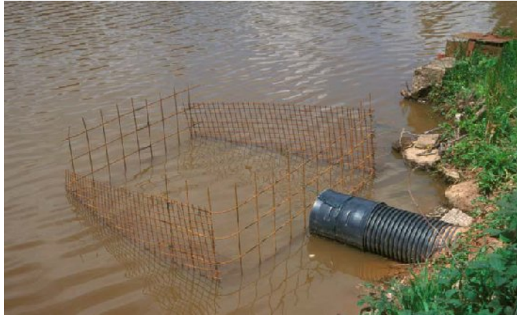
Photo No. 43.: Protection of an outflow pipe from a fish pond with wire grating.
