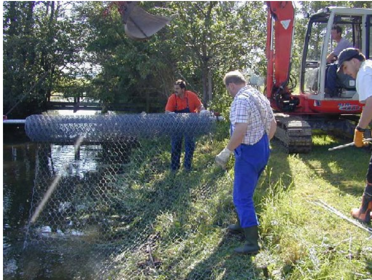
Photo No. 45.: Bank revetment with a wire grid
