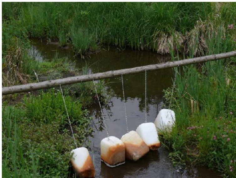
Photo No. 42.: Not an optic beauty, but simple and cheap: some plastic canisters above the creek prevent rebuilding of a beaver dam
