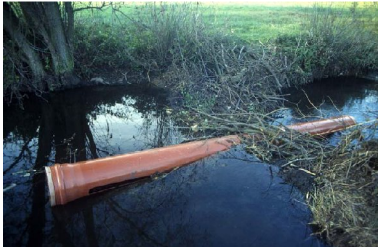
Photo No. 41.: A flow device (here with a 40 cm pipe) creates a compromise between water level required by beavers and acceptable by land users
