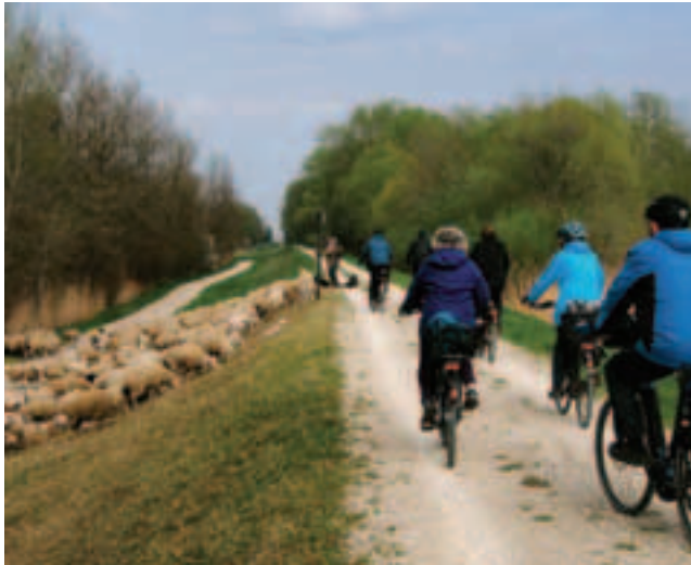
Grazing is important to keep dam sides in good condition. And herds consisting of sheep and goats (like this one) are an especially efficient tool: sheep cut the higher grass while goats do fine trimming, eating what is close to the ground.
